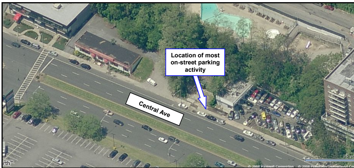
Figure 5: Southbound Central Park Avenue On-Street Parking north of Fort Hill Road
