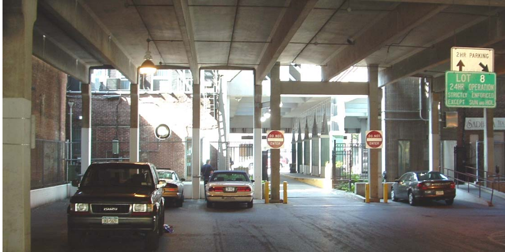
Fig. 13 – This is a view of the interior of the Third Street Garage interior looking out toward the Gramatan Avenue entrance.
