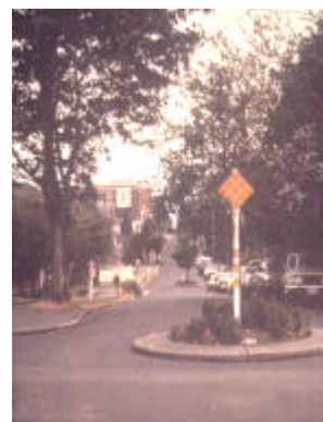
Traffic circles and other devices such as textured surfaces, raised intersections and neckdowns are techniques that reduce vehicle speeds and help manage traffic in downtowns and on local neighborhood streets.
