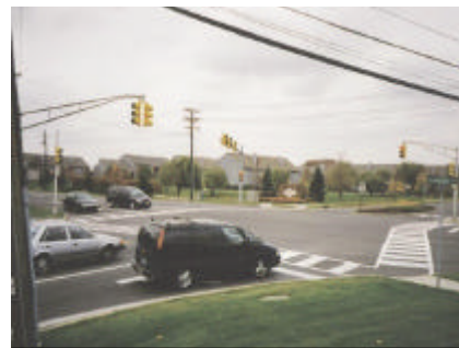
Crosswalk treatments may include diagonal or longitudinal lines for added visibility, especially at high-volume pedestrian crossings and at mid-block.
