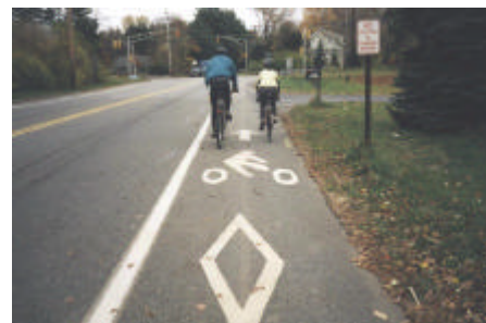
Bike lanes are appropriate facilities on arterials and major collectors, with the following advantages: They help to define road space, provide an obstacle-free path, reduce stress and give cyclists a right to the road.
