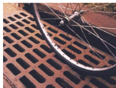
Bicycle-safe drainage grates prevent narrow bicycle wheels from being trapped between grate openings.
